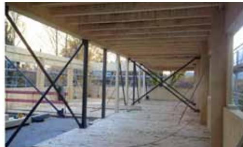
6 | view of the building site while putting up the wood columns of the ground floor
